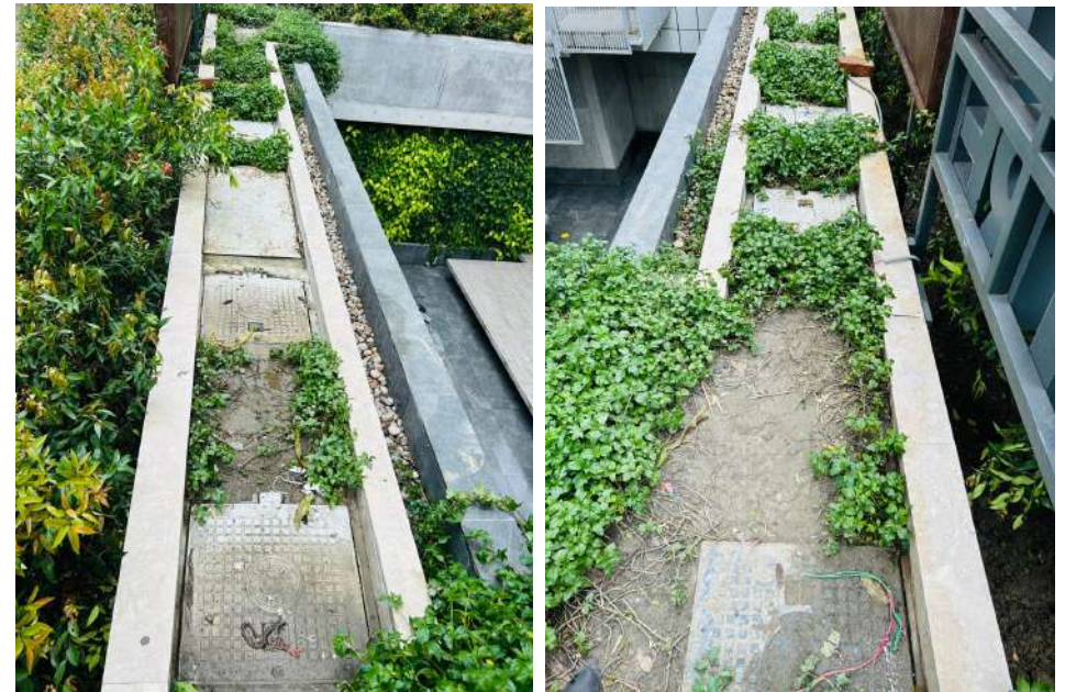
Sewage Treatment Plant - MBBR Technology
