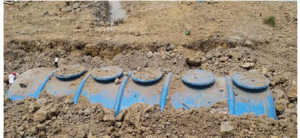
Sewage Treatment Plant
